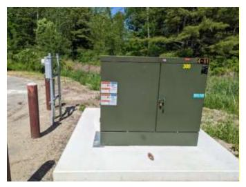
Figure 9 Dedicated Transformer for BEB Chargers at 13 Pomerleau St.
